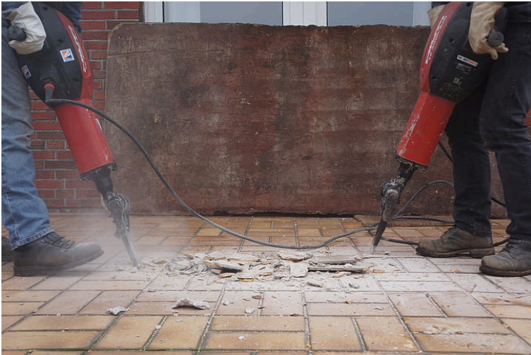
Figure 9.6: Two workers jackhammering a hard floor
