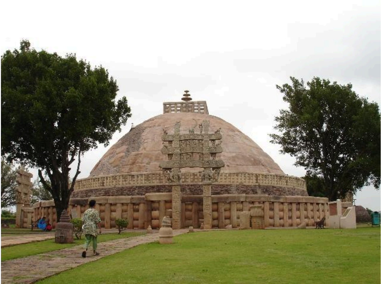
Figure 11.13: Mauryan and later Maker(s) of Sanchi, India. Mahastupa . ca. 50 BCE – 400 CE. Brick and stone masonry, 106' diameter x 42' tall. In situ. CC BY-SA 1.0 .
