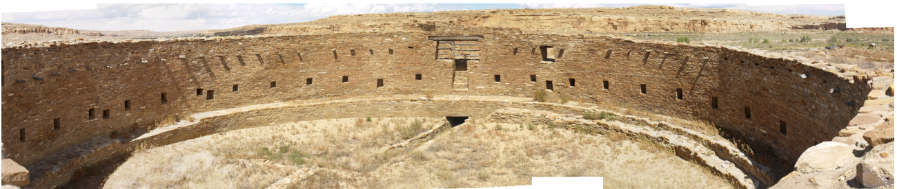
Figure 7.7: Ancestral Puebloan Maker(s) from Chaco Canyon, New Mexico. Kiva of Casa Rinconada . ca. 1050-1150 CE. Masonry, 64' diameter. Merged panorama by Leah McCurdy; CC BY-NC-SA 4.0 .
