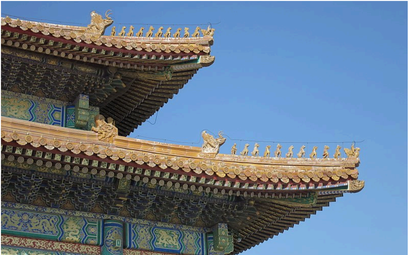
Figure 13.3: Detail of roof system at the Taihedian . Photo by 秋水平湖; CC BY-SA 3.0 .
