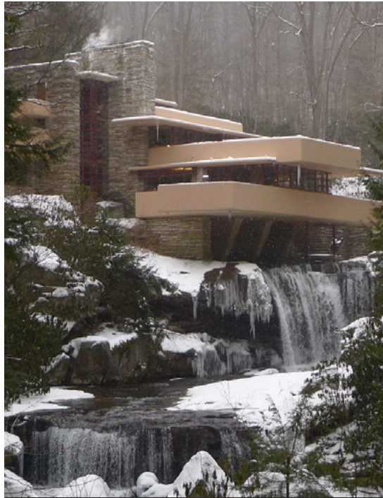
Fig.02/04 The concrete cantilevers in Fallingwater House sets a stark contrast with nature.
