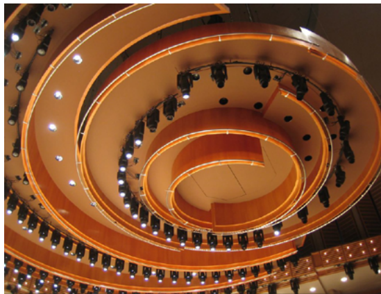
Fig.03/18 Curved wood paneling in this concert hall ceiling is used to direct and diffuse the sound.
