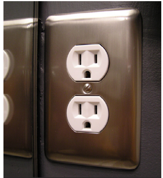
Fig.03/08 An example of user tolerance, the typical electrical outlet features one slit slightly longer than the other, so the plug is inserted correctly every time.
