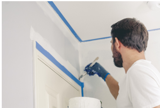
Fig.05/16 Painting is a messy process, and masking is a requirement for even the smallest job.
