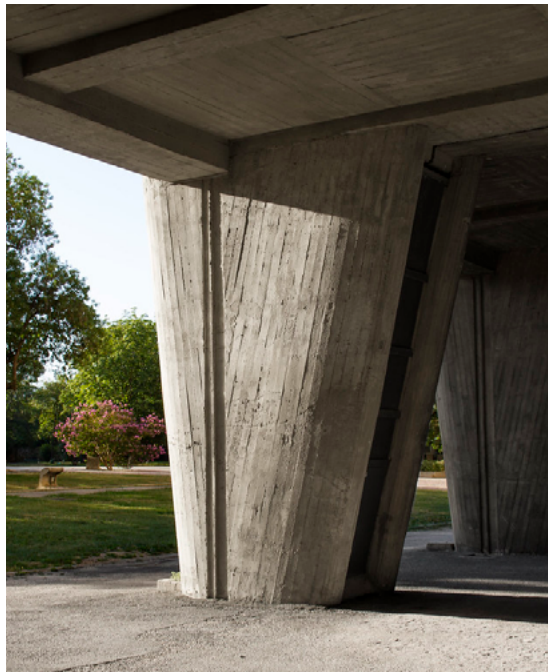
Fig.02/03 Brutalist architecture features substantial amounts of unfinished concrete surfaces.
