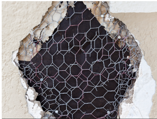
Fig.05/13 Laborious to install, a furred diamond wire lath provides good basis for plaster to hold on.
