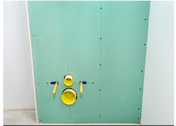
Fig.05/10 Green-board is appropriate where some moisture exposure is expected.
