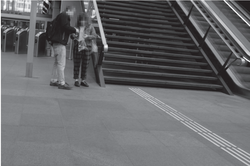
Figure 9.12b Showing a segment of tactile paving within the terminal building of The Hague central station.
