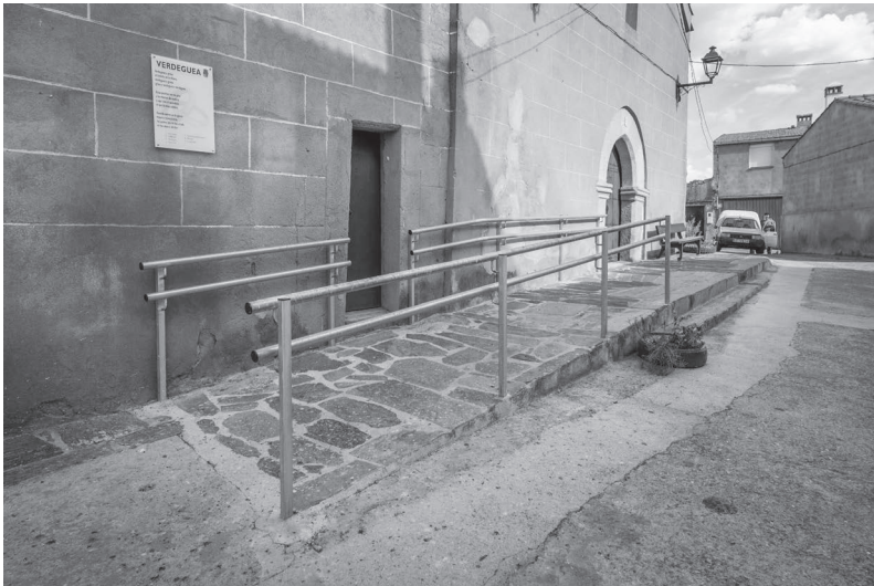
Figure 10.20 Safe route (above) and handrails at the church access (below).
