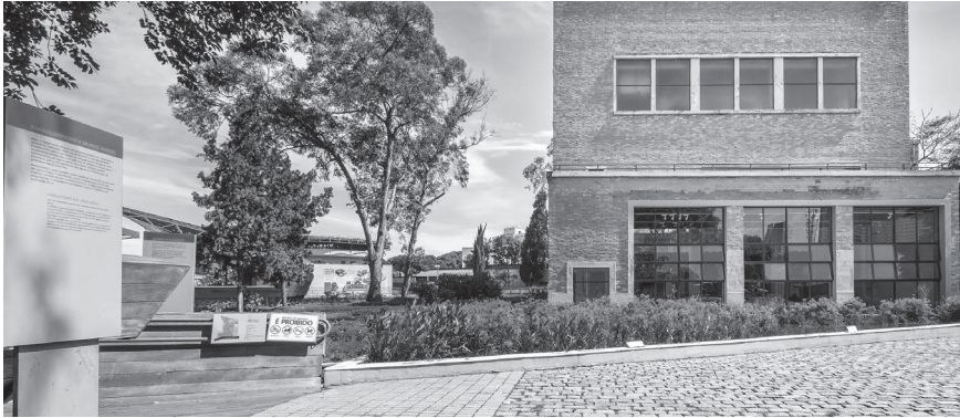
Figure 10.47 The old incinerator building and the informational stations.
