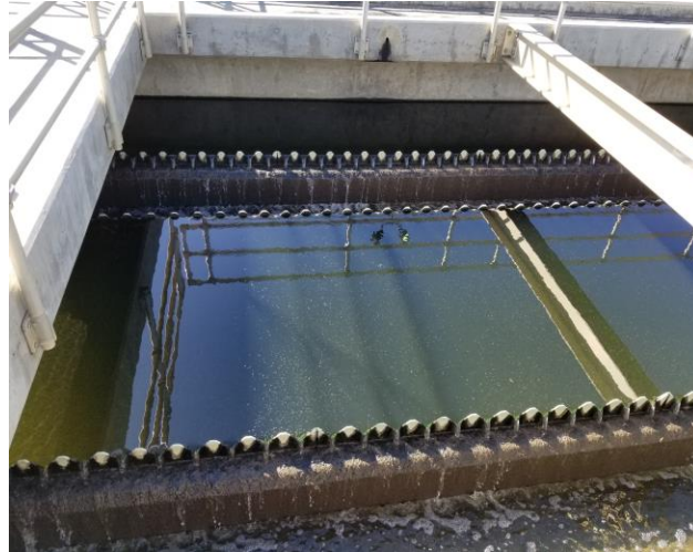
Figure 5.2: Sharp crested weir 27
