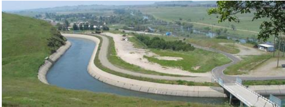
Figure 2.7: Public Domain from U.S.G.S. of California Aqueduct through the Central Valley transporting water from Northern California to Southern California 7
