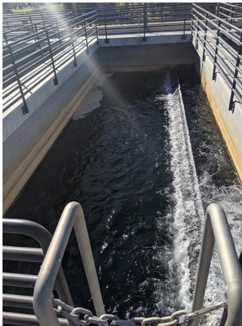
Figure 5.3: Broad crested weir 28
