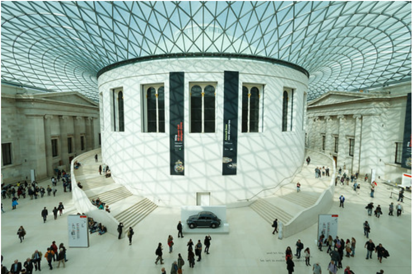
Figure 5-8: The free form of the space frame that covers the British museum courtyard ((Image source: British Museum, 2014, https://www.flickr.com/photos/22087304@N07/15629080951 )
