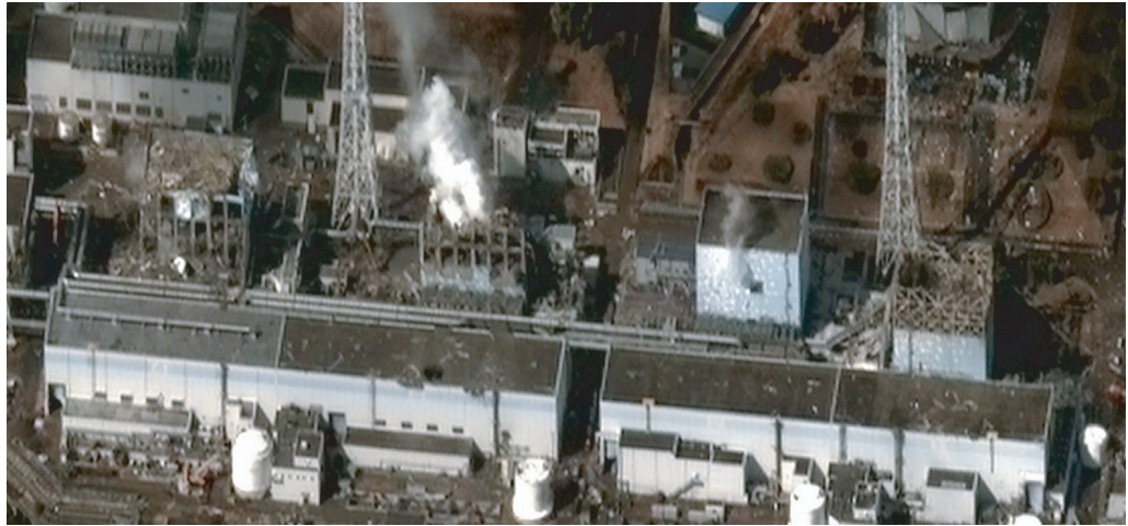
FIGURE 111 The destruction of four nuclear reactors in 2011 in Fukushima, in Japan, which rendered life impossible at a distance of 30 km around it (courtesy Digital Globe).
