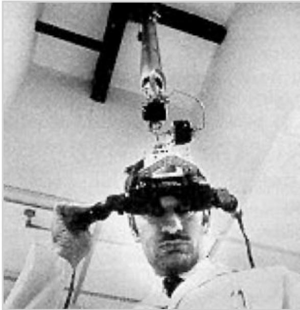
The ultrasonic head position sensor
