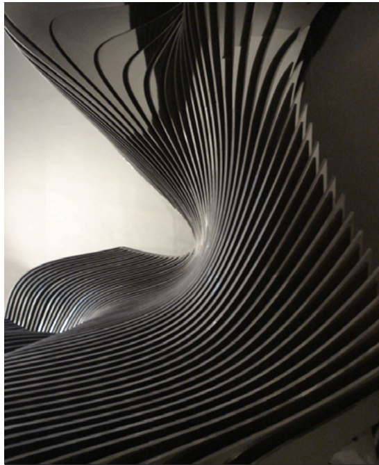
Fig.07/43 MDF panels can be CNC cut, lacquered, and installed in a sequence to define complex curves.
