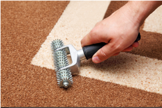
Fig.09/34 A grooming roller can be used to improve the performance and look of the seam.
