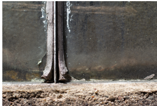
Fig.08/14 Glass sealers can dry in the long term, losing resiliency and starting to peel off.
