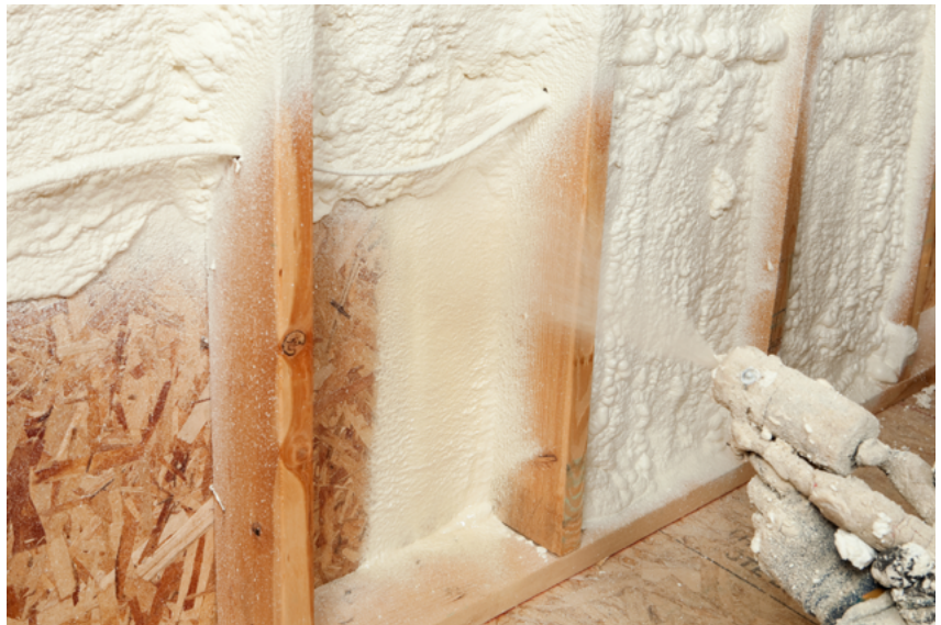
Fig.11/20 Polyurethane spray-foam insulation is highly efficient but requires flawless installation to properly function.
