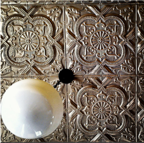
Fig.10/25 Embossed tin ceiling tiles can retain intricate detail and introduce a unique sheen.
