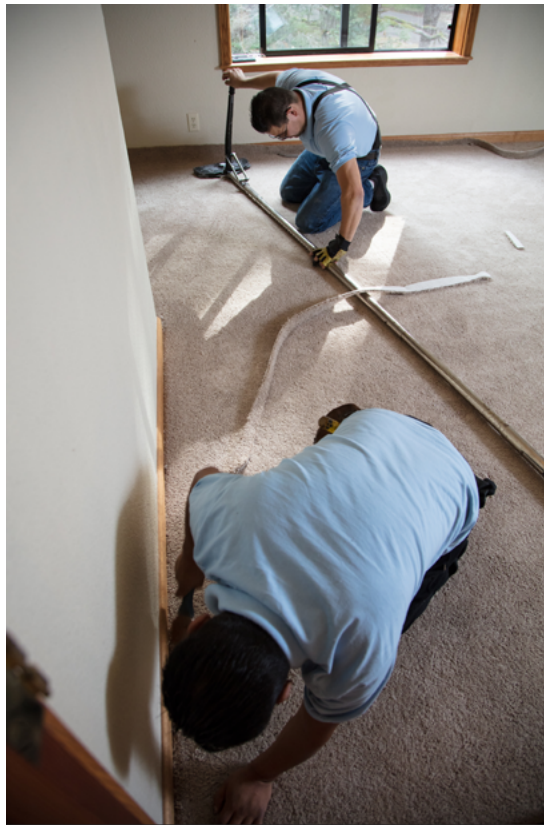
Fig.09/32 The long tool is the power stretcher, a crucial tool for stretch-in installation process.
