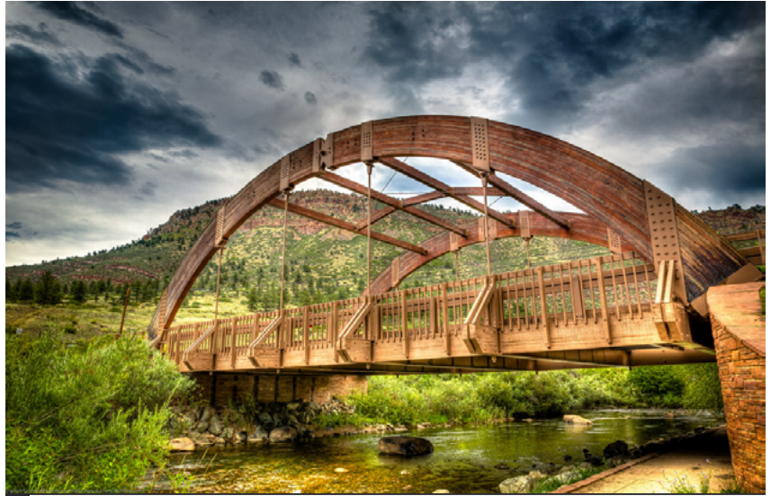
Fig.07/42 The Apple Valley Road Bridge in Lyons, CO utilizes bent GluLam beams as the structural component.
