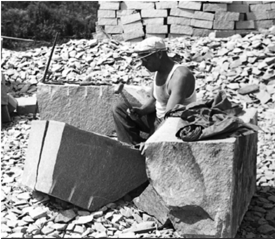
Fig.06/17 A 1936 photograph from a Maine quarry depicting how the stones were manually processed.
