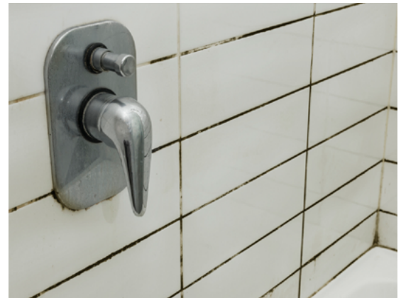
Fig.03/11 Black mold can be fairly inconspicuous sometimes appearing as dirt or stain.
