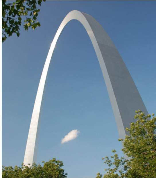
Fig.10/02 304 series stainless steel alloy panels were used for the Gateway Arch construction.
