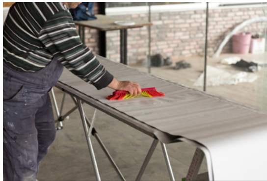
Fig.05/23 Adhesive is being applied on cut strips of wallcovering.
