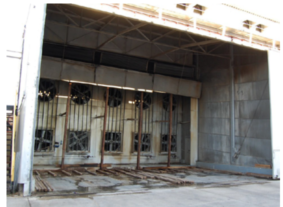
Fig.07/28 Lumber drying kiln.
