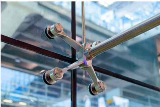
Fig.08/13 Glass panels can be suspended with spider fittings, enabling a continuous look without mullions.
