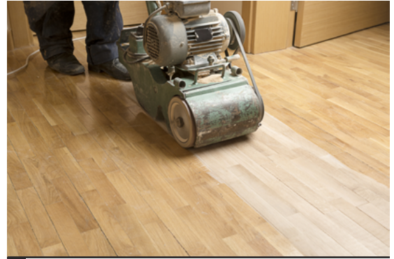
Fig.07/34 Solid wood and veneer can be sanded and refinished multiple times.
