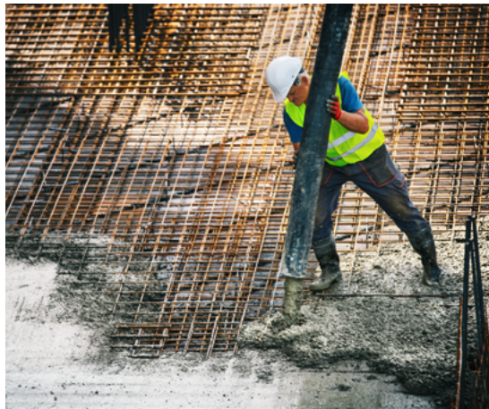
Fig.01/11 Concrete mixture poured over rebar lattice.
