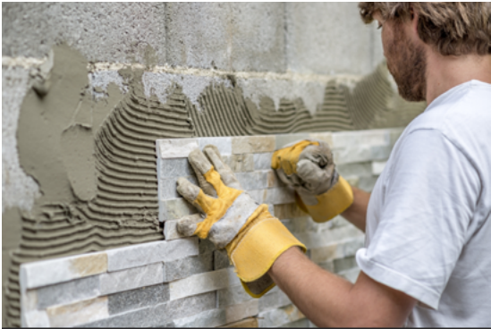
Fig.06/25 Natural stone veneers are being thinset on CMU (Concrete Masonry Unit) wall.
