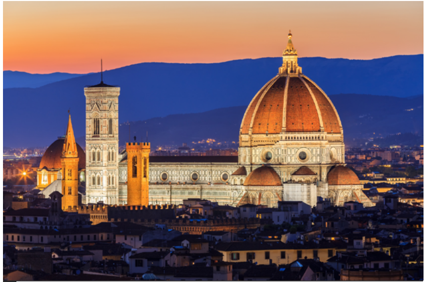
Fig.06/10 Constructed in 1420, the masonry dome of Santa Maria Del Fiore in Florence, Italy spans 144 feet.
