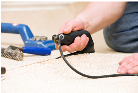
Fig.12/08 Seaming iron is one way to join carpet seams. More seams mean more labor and increased cost.
