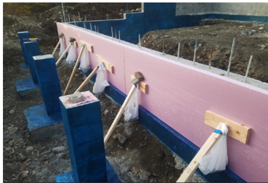
Fig.11/15 The pink colored extruded polystyrene (XPS) is a common insulation material.
