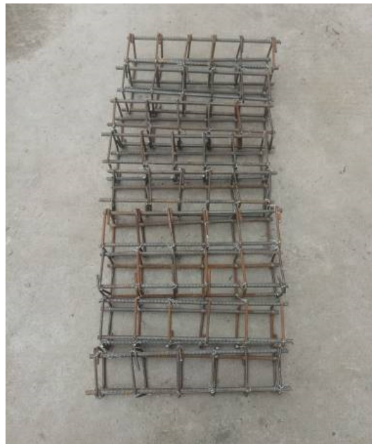
Figure 5. The reinforcement of the short column.
