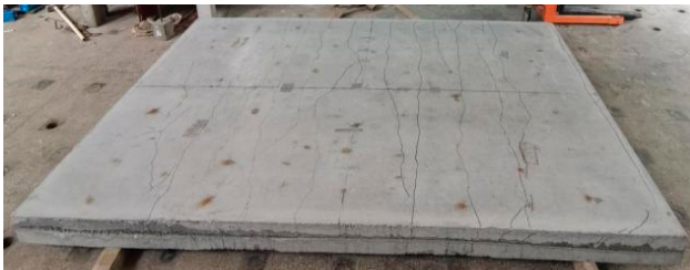
(a) Crack distribution at slab bottom
