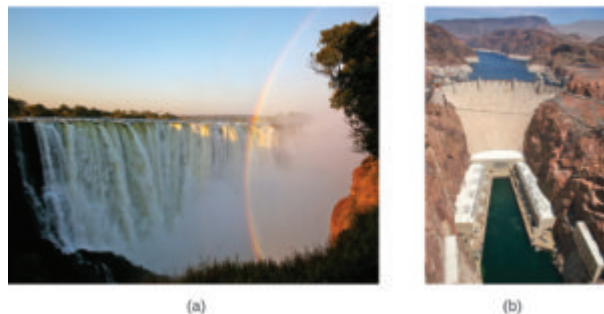
Figure 2 (a) Water that is higher in elevation, for example, at the top of Victoria Falls, has a higher potential energy than water at a lower elevation. As the water falls, some of its potential energy is converted into kinetic energy. (b) If the water flows through generators at the bottom of a dam, such as the Hoover Dam shown here, its kinetic energy is converted into electrical energy. (credit a: modification of work by Steve Jurvetson; credit b: modification of work by “curimedia”/Wikimedia commons)
