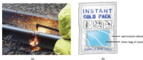
Figure 6 (a) An oxyacetylene torch produces heat by the combustion of acetylene in oxygen. The energy released by this exothermic reaction heats and then melts the metal being cut. The sparks are tiny bits of the molten metal flying away. (b) A cold pack uses an endothermic process to create the sensation of cold. (credit a: modification of work by “Skatebiker”/Wikimedia commons)
