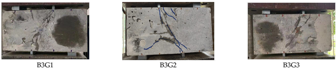
Figure 8. Shear damage with different spacing of bars.
