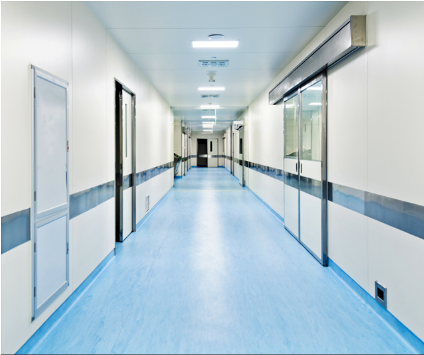
Fig.11/11 Vinyl flooring application in an operation room corridor, the welded seams and flash coving at the perimeter are compatible with the strict hygiene require-
