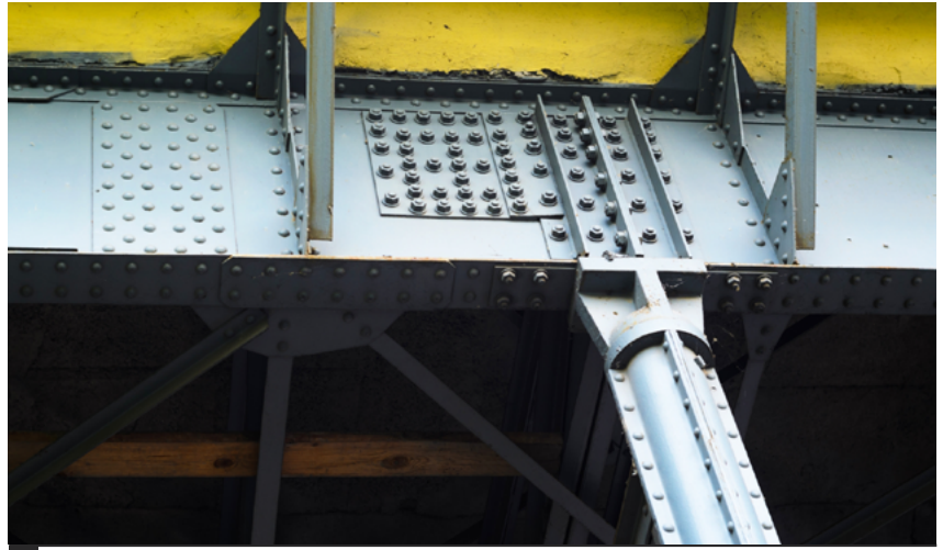
Fig.10/08 Riveting is a time consuming process, harder to conduct on-site, therefore a mixture of rivets and bolts is not an uncommon sight in construction.
