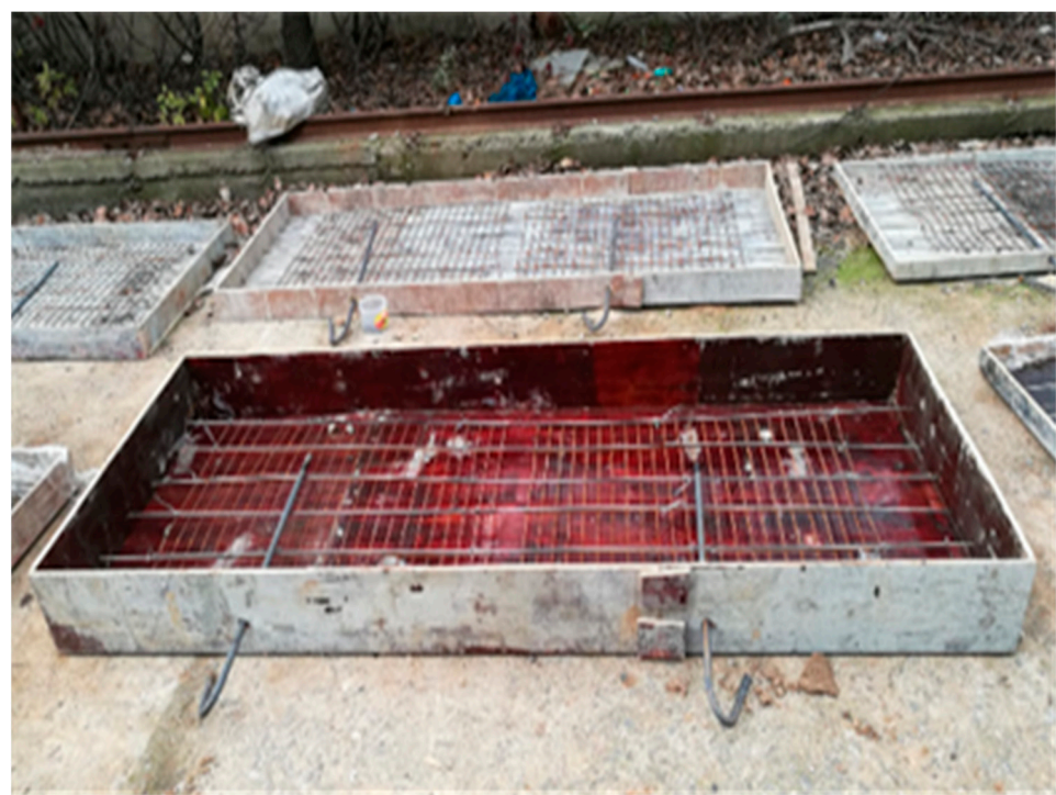
Figure 4. Mold making and steel binding.
