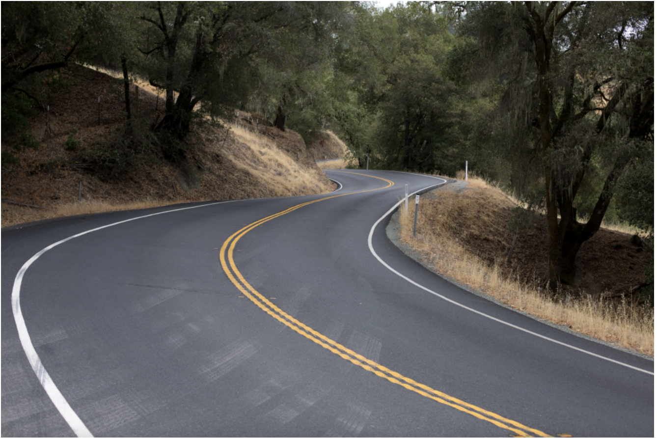
Figure 2: "Curvy road." No author. (CCO)
