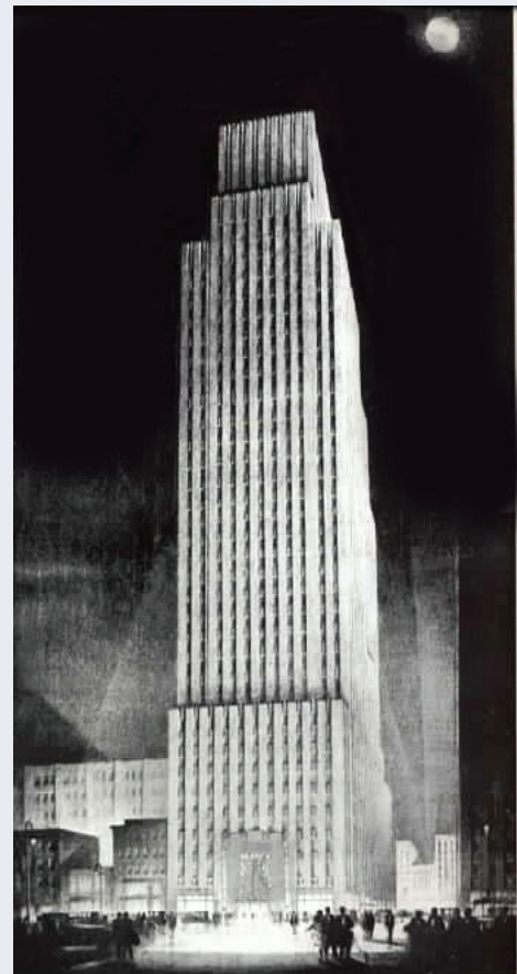
Figure 2.45 | New York Daily News Building
