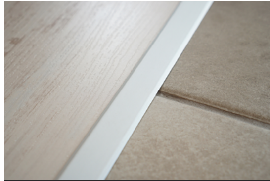
Fig.09/35 Trim strips conceal the seam between two different flooring materials.
