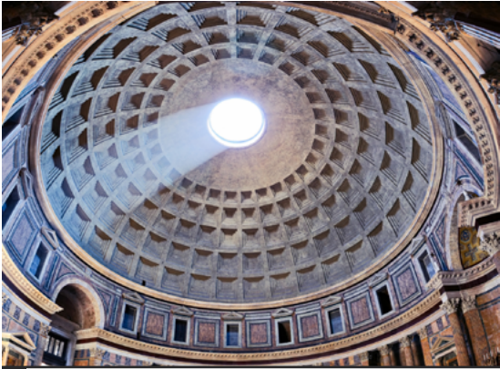
Fig.06/01 The dome of Pantheon showcases the capabilities of concrete as a construction material.
