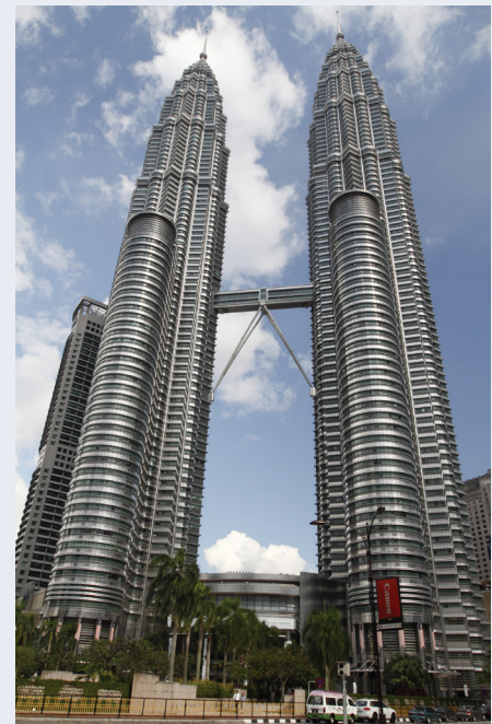
Figure 7.38 | Petronas Twin Towers, Malaysia
