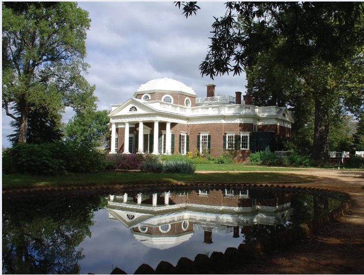
Figure 7.19 | Monticello, Charlottesville, VA
