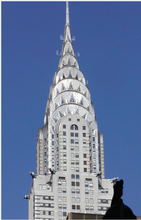
Figure 7.37 | The Top of the Chrysler Building, New York City, NY
