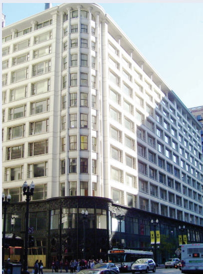
Figure 7.34 | Carson, Pirie, Scott and Company Building, Chicago, IL
