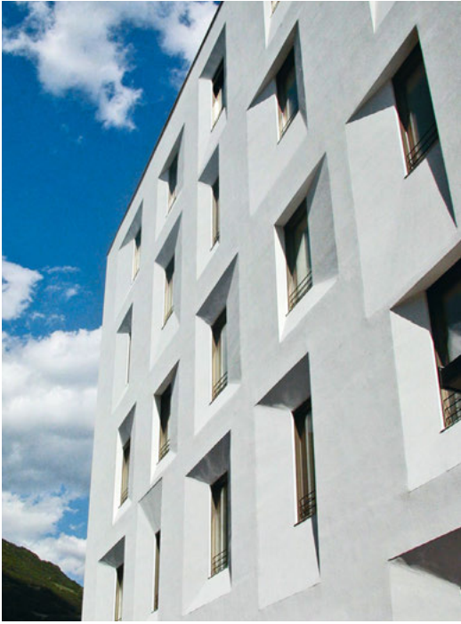
Fig. 2.10: 'Expost' office refurbishment project, Bolzano. Angled window reveals serve as an architectural design element while keeping good daylighting and unobstructed views to the outside despite thick exterior insulation.
