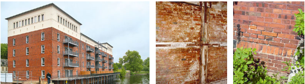
Fig. 6.2: Warehouse City Building in Potsdam, a timber-framed construction, open joints on the outer facade
