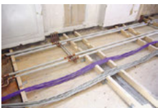
Fig. 4.10: New piping and cables under the floor
