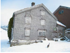
Fig. 8.3: East (above) and west facade (bottom)
