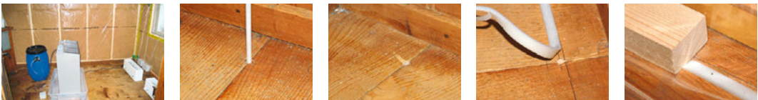
Fig. 8.6: Installation of the internal insulation
