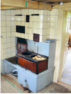
Fig. 3.11: Strickbau Appenzell (CS8), wood fired stove in the kitchen, backed by a tiled stove on the other side of the shared wall. Heating takes a central position in the building.
