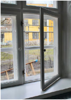
Fig. 4.7: New coated glass, inside frame
