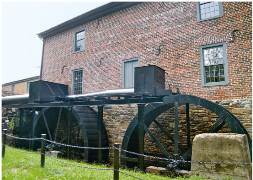
Fig. 5.71: Historic mill utilised for a modern hydroelectric scheme
