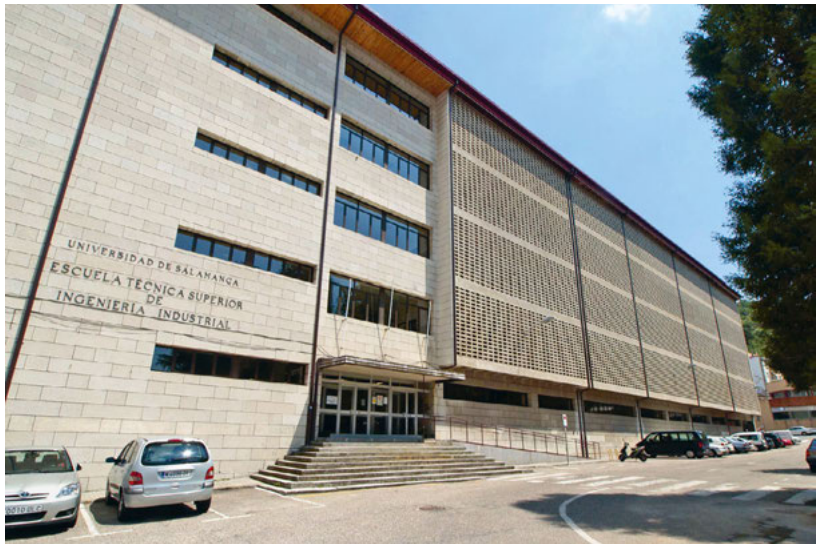
Fig. 7.1: Main facade of the building
