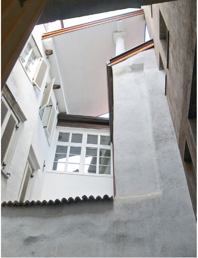
Fig. 3.15: Atrium, enabling subdued light and ventilation for the internal rooms, Bolzano, Italy
