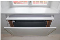
Fig. 4.9: Cooling and heating by convectors
